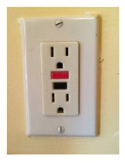
Note that the outlet to the right of the sink becomes energized when the light switch is on (and it is also protected by the GFI outlet).
